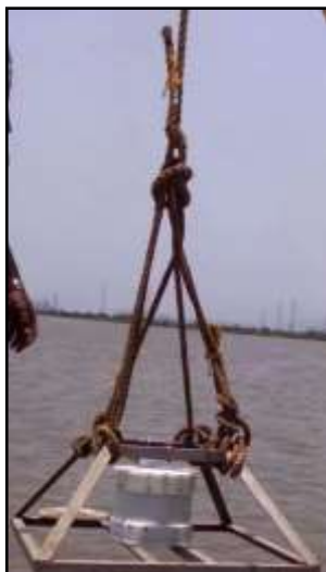
Fig. 5a: Lifting of Tide gauge & metal frame using winch.
